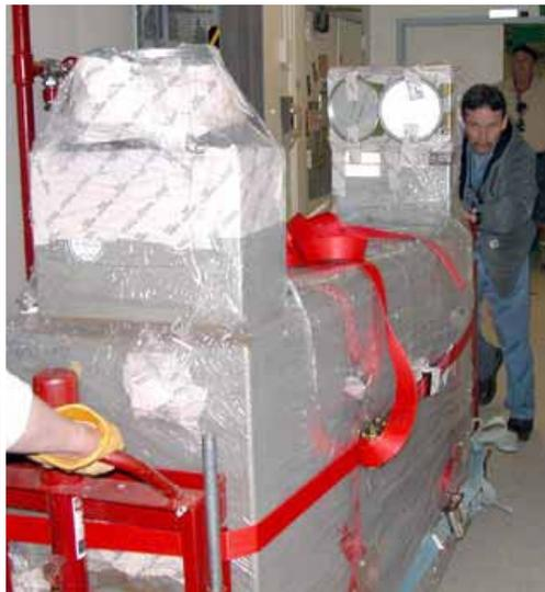
The D&D workers at the Plutonium Finishing Plant are making progress within the 234-5Z Building, a former plutonium processing facility. Glovebox removal continues ahead of schedule so that demolition of the facility can be accelerated.
