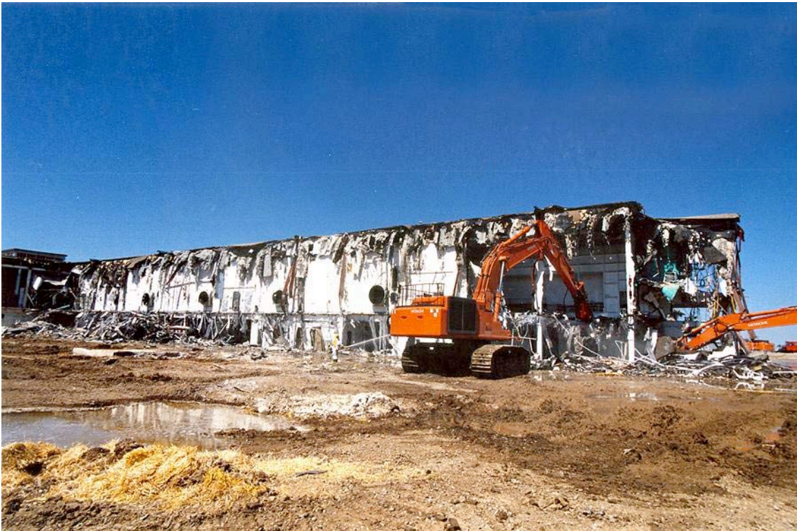
Building 776/777 Demolition is Approximately 60 Percent Complete
