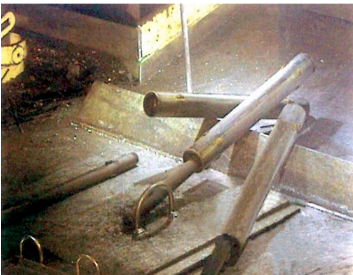
Spent Fuel in Fair Condition
