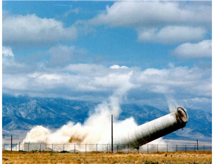
Engineering Test Reactor Exhaust Stack Demolition
