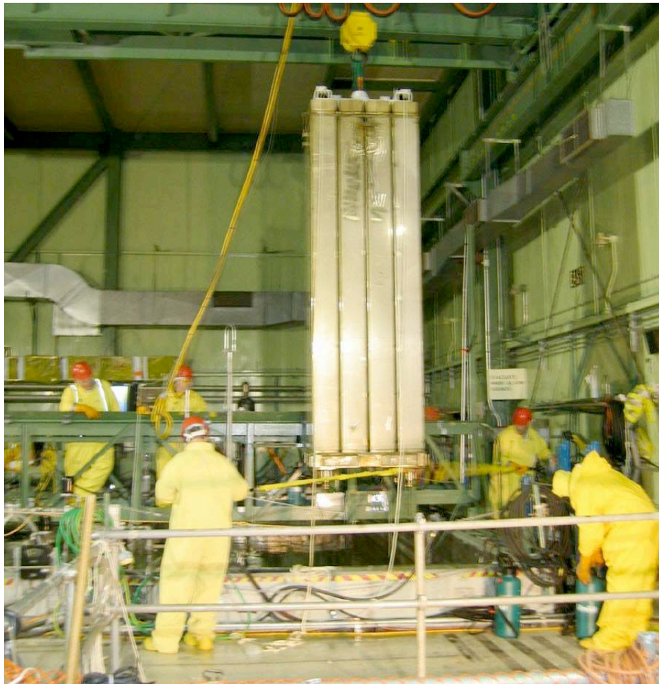
Connecticut Yankee Fuel Rack Removal
