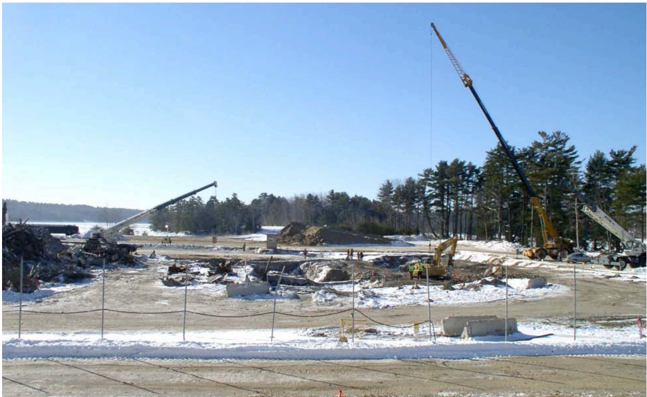
General View of Yard Area of Former Maine Yankee Power Plant
