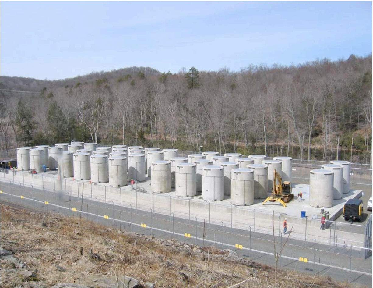
Connecticut Yankee Final Spent Fuel Storage – 43 Casks
