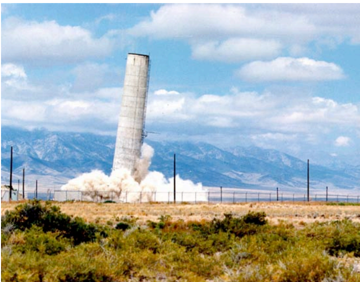
Engineering Test Reactor Exhaust Stack Demolition
