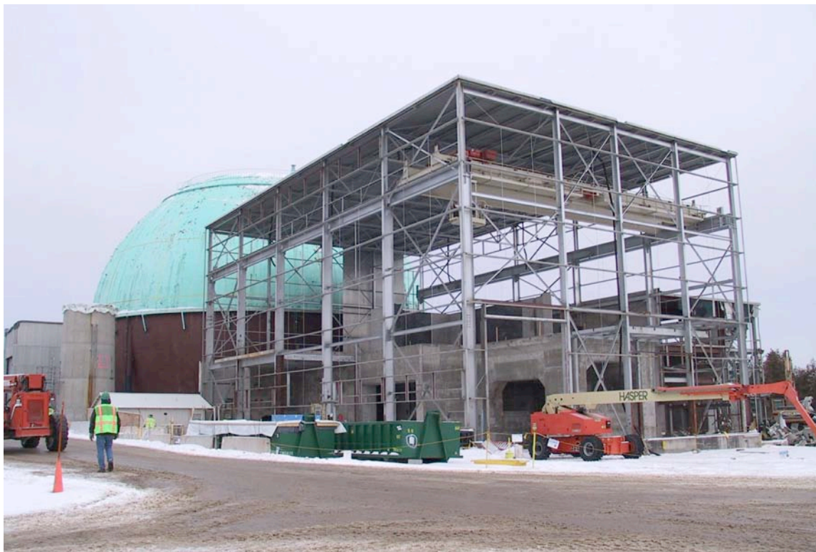
Three Story Turbine Building Stripped of Steel Panel Walls Prior to Demolition
