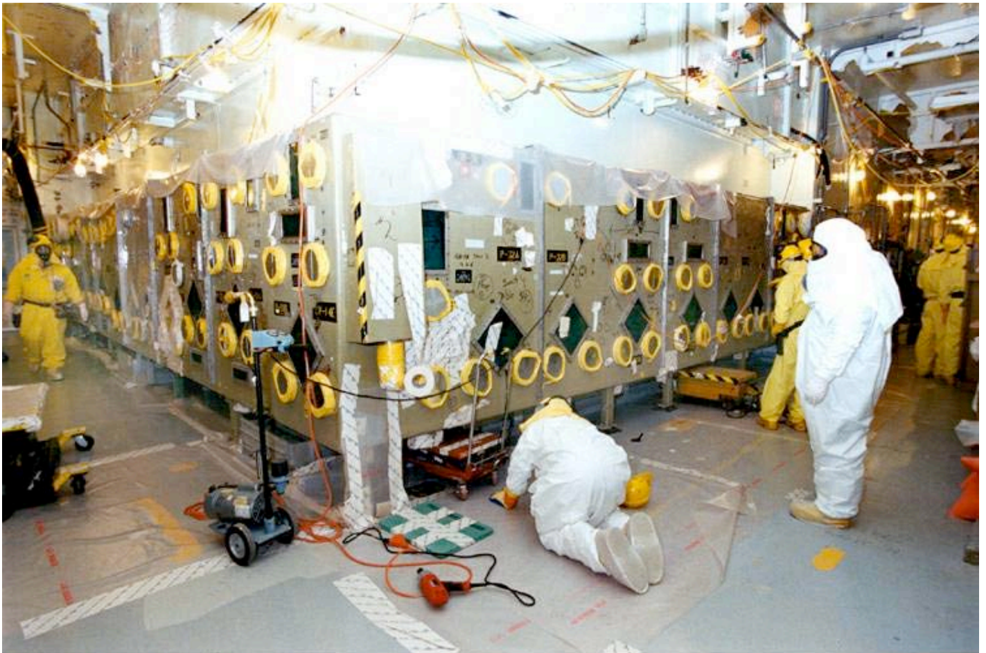
Workers Prepare to Remove the last of 1,457 Glove Boxes from Building 371
