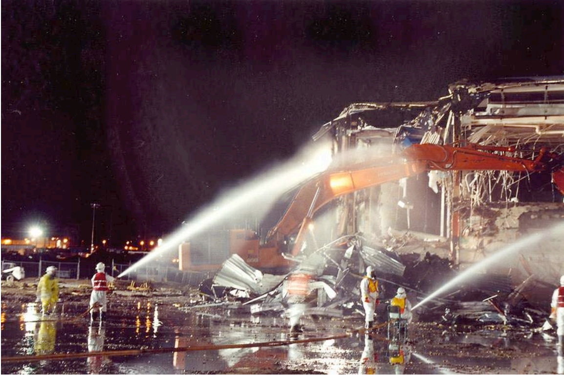
Spraying Water for Dust Suppression during demolition of Building 776/777
