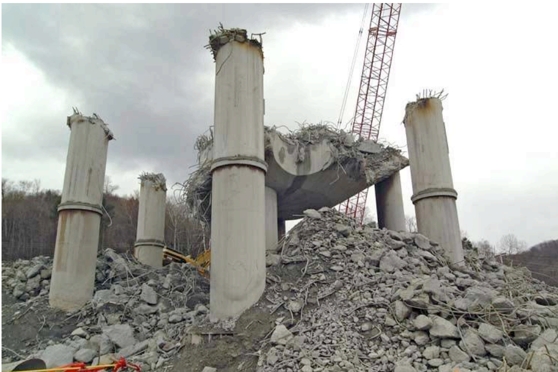
The Reactor Support Structure as it remains in April 2005
