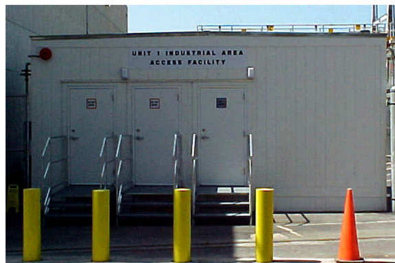
Unit 1 Industrial Area Access Facility
