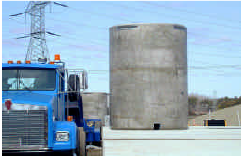
M-Y Empty Vertical Concrete Canister Placed on Pad
