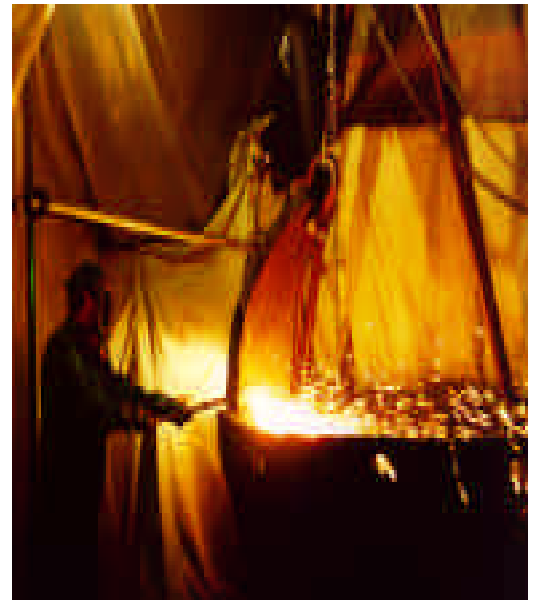
Cutting Up Sodium Pentaborate Tank
