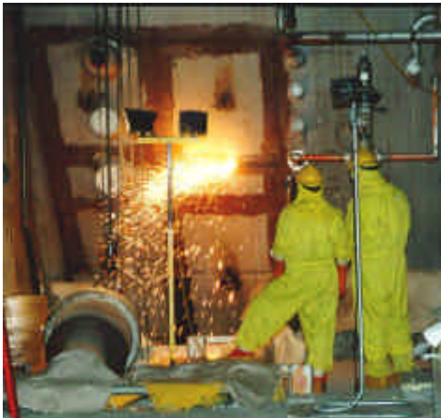
Cutting Hole in Containment Sphere
