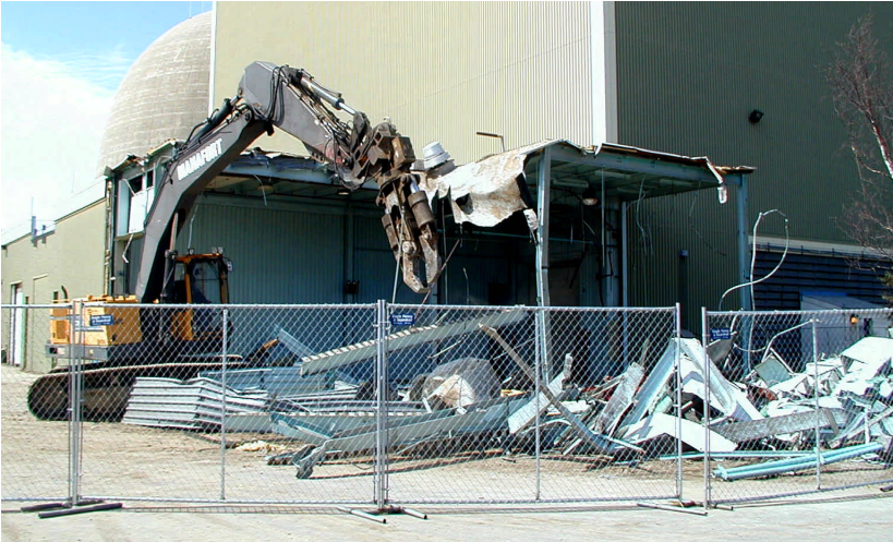
Demolition of M-Y Turbine Building Cool Side Machine Shop
