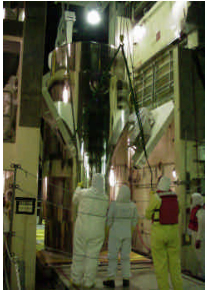
The Spent Fuel Transfer Cask after removal from Pool
