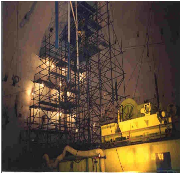
Final survey of the Containment dome was safely performed using scaffolding built on top of the polar crane 150 feet in the air.
