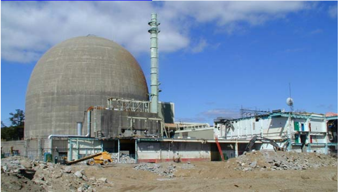
View of Containment and Remaining Turbine Building Structure (April 2002)
