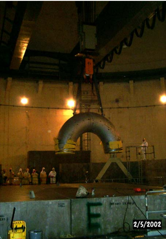
Removing the First Section of Reactor Coolant Piping
