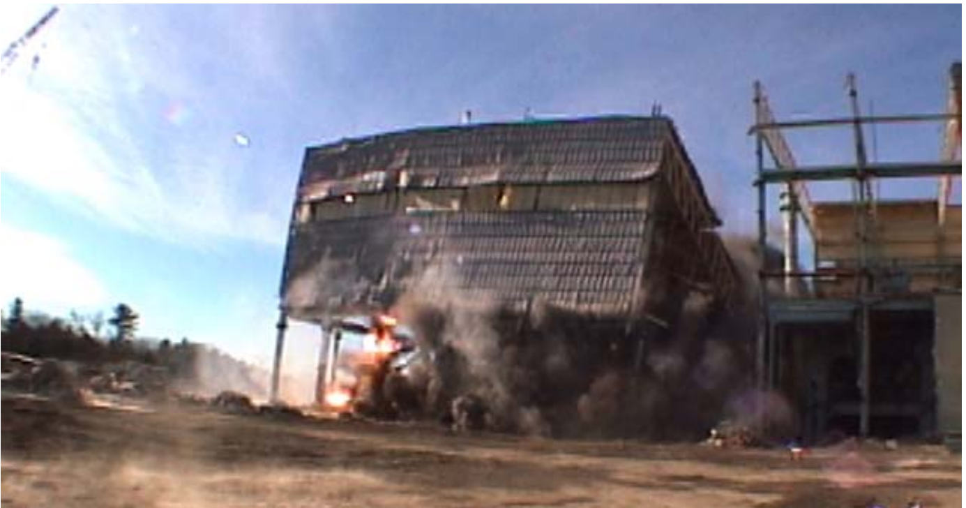
Turbine Building Implosion (November 2001)
