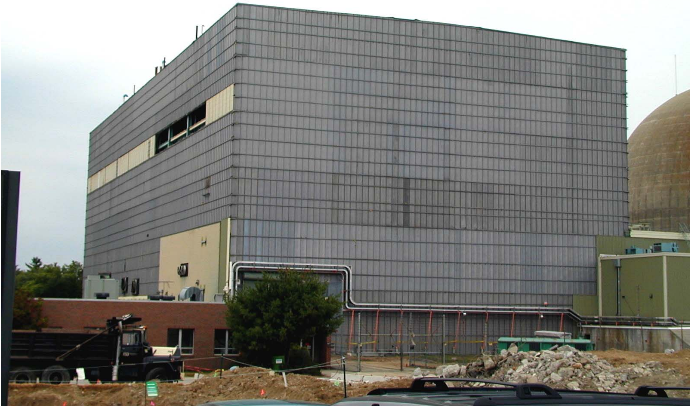
Turbine Building With Siding Removed (August 2001)
