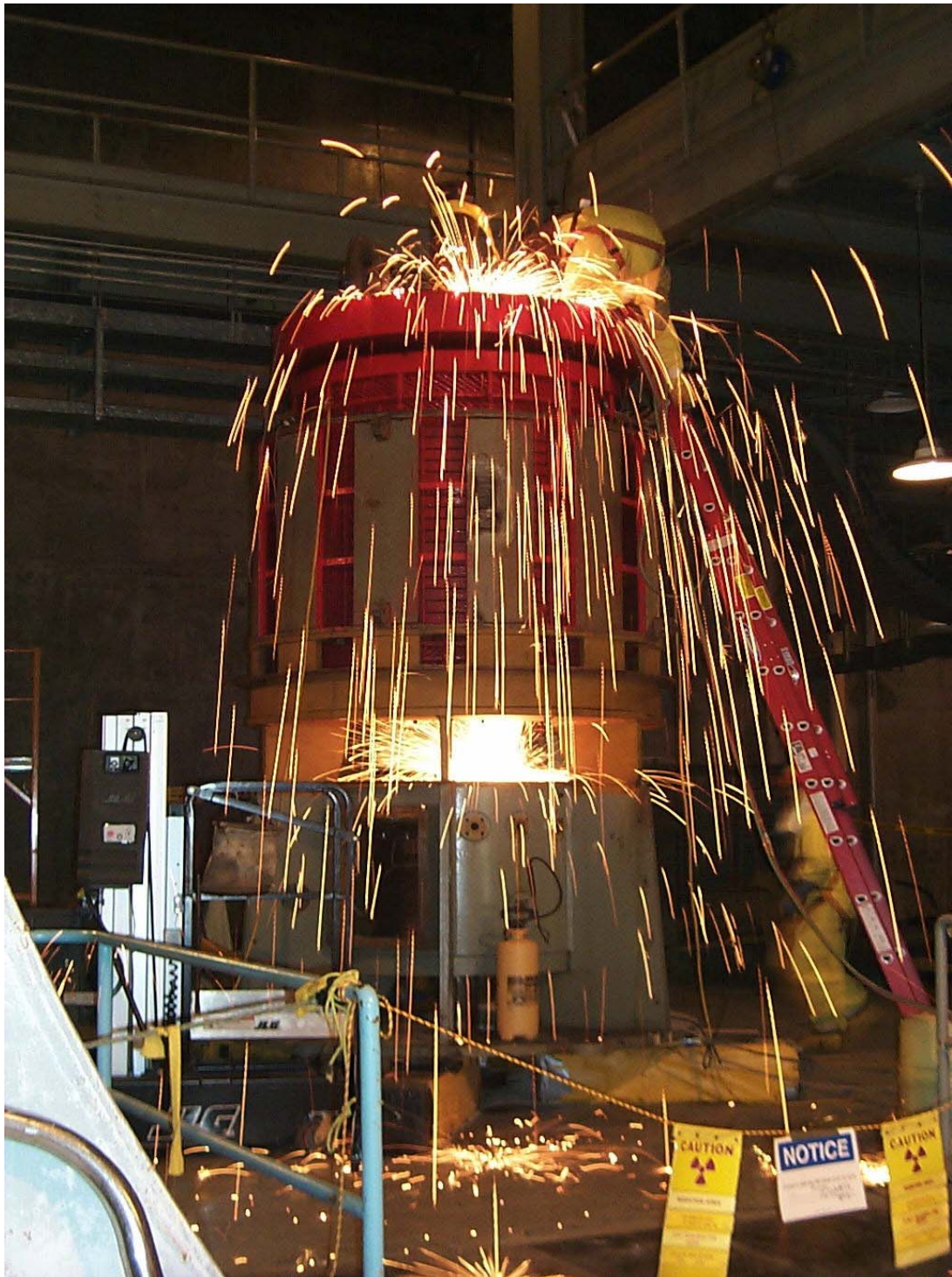
Cutting Up a Reactor Coolant Pump Motor
