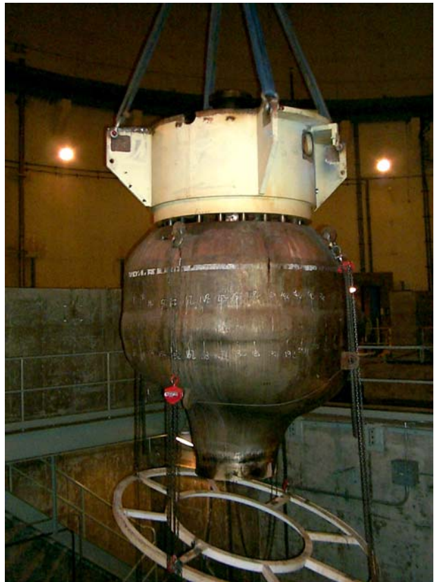
Removing the First Reactor Coolant Pump
