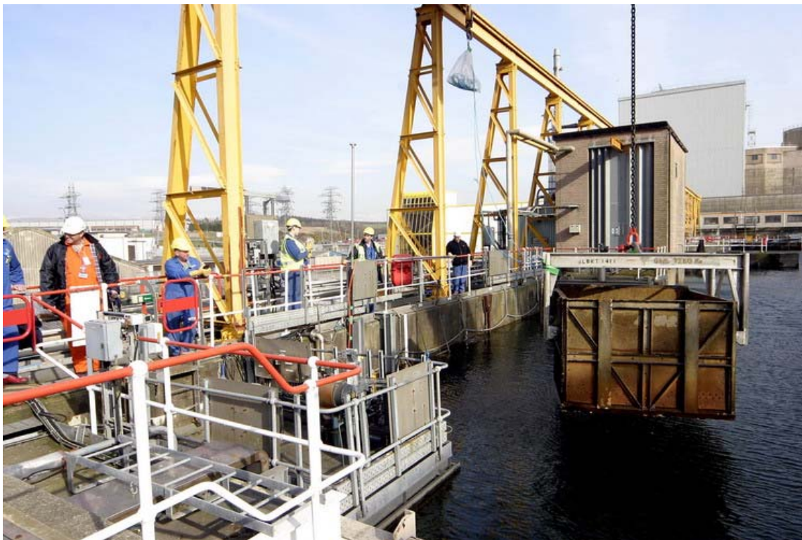
The first skip in 6 years is removed from the Pile Fuel Storage Pond
