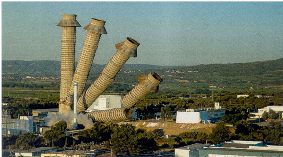
Explosive dismantling of the G-1 reactor stack in France
