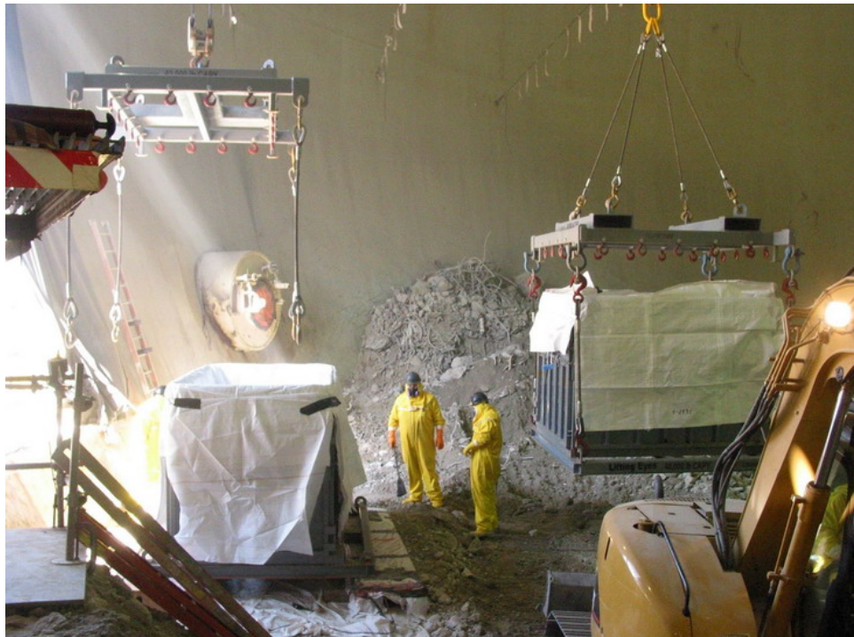
Containment loading lift liners for removing crushed debris
