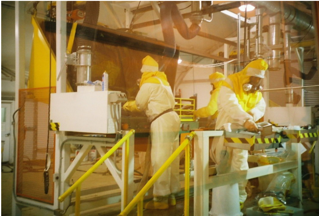
Workers process waste in one of the WVDP's waste processing containment structures
