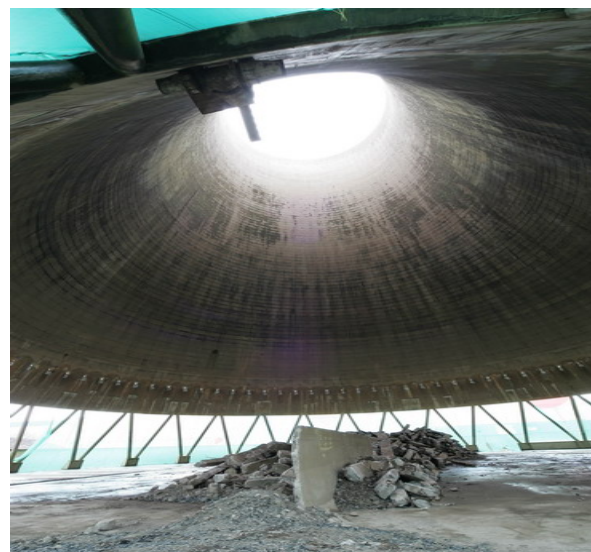
Removal of internal material from the Calder Hall Cooling Towers
