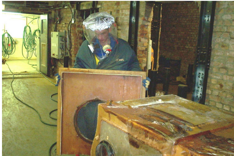
A worker dismantling an alpha contaminated glove-box at the North Group Compound
