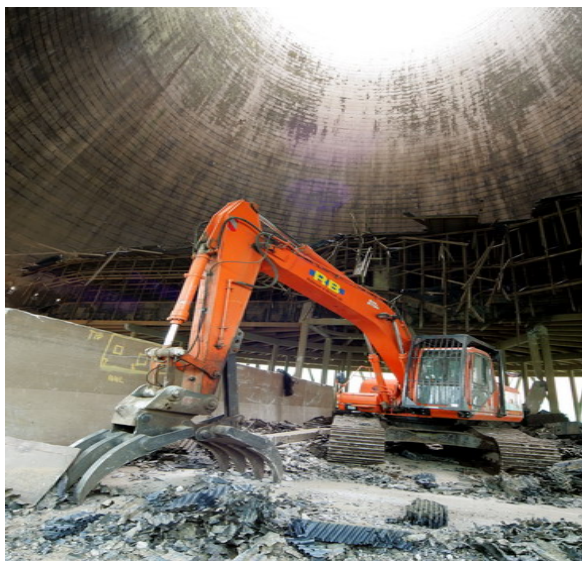
Removal of internal material from the Calder Hall Cooling Towers
