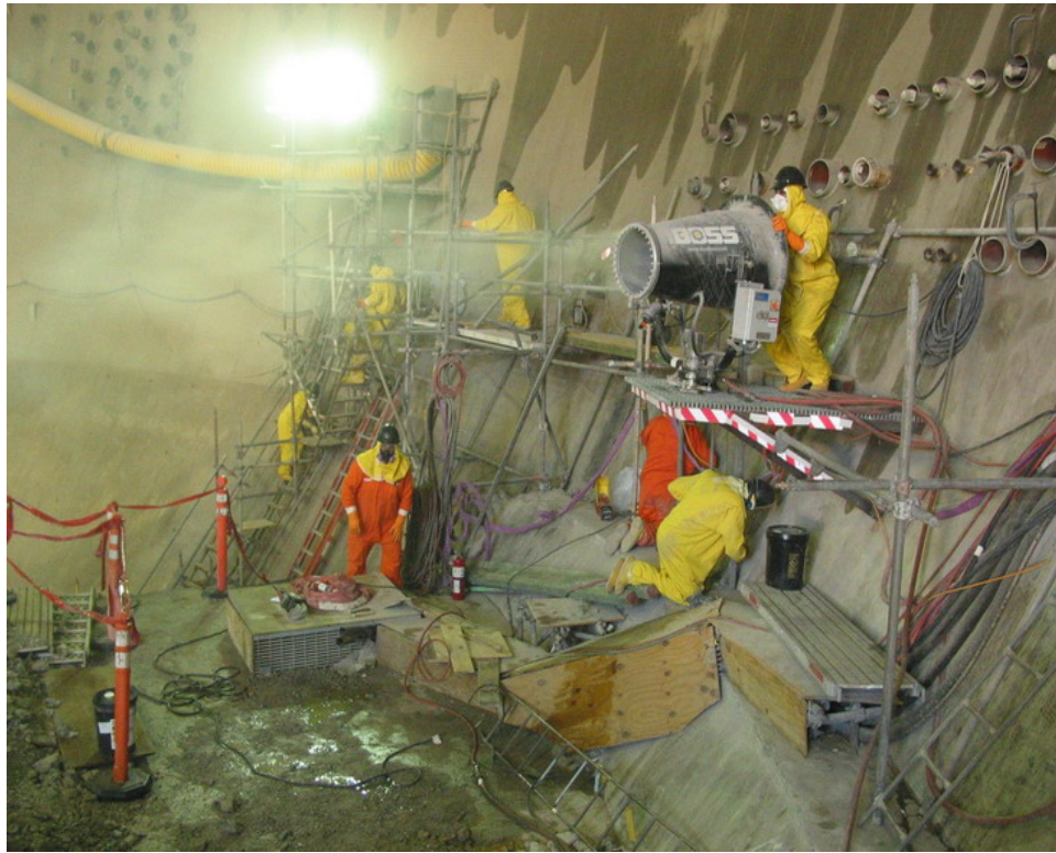
Photo inside containment using fog canon to control demolition dust
