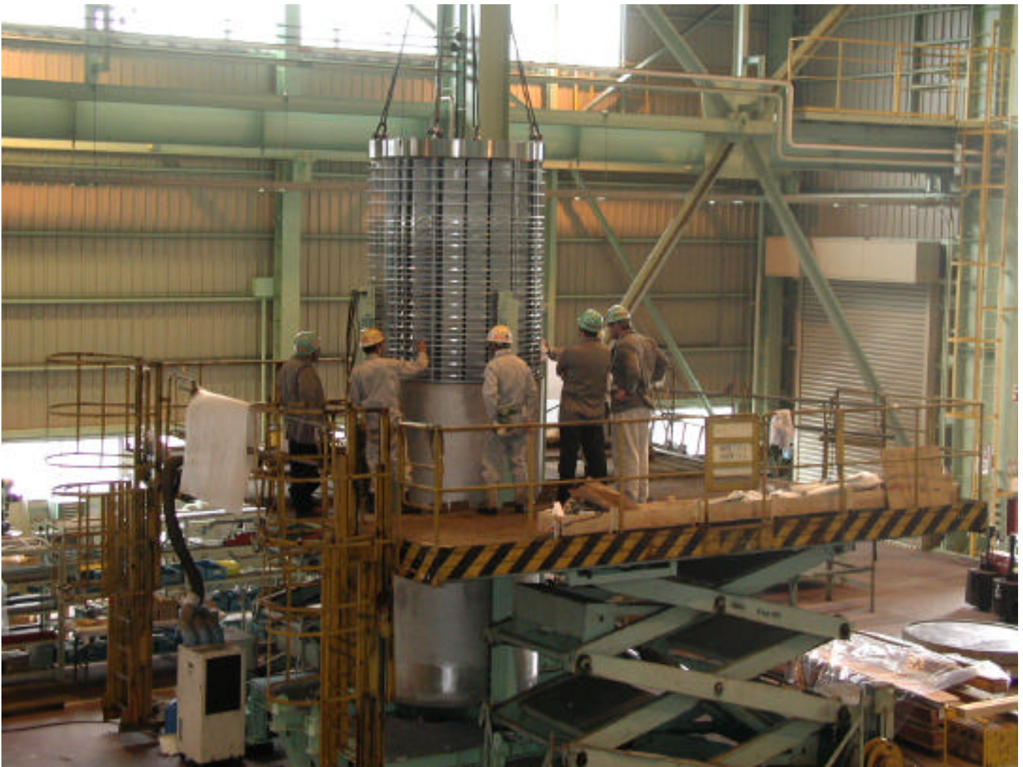
Basket Being Inserted into Canister during Canister Fabrication at Hitachi Zosen in Japan
