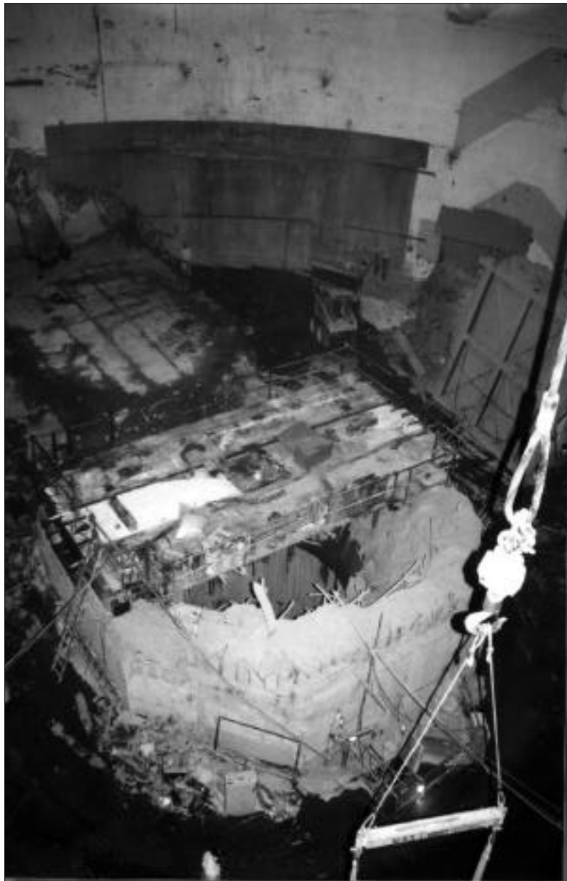
Remaining Reactor Cavity within the Trojan Containment Building
