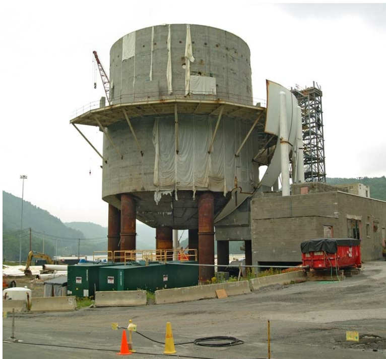
View of Reactor Support Structure after removal of Vapor Container.
