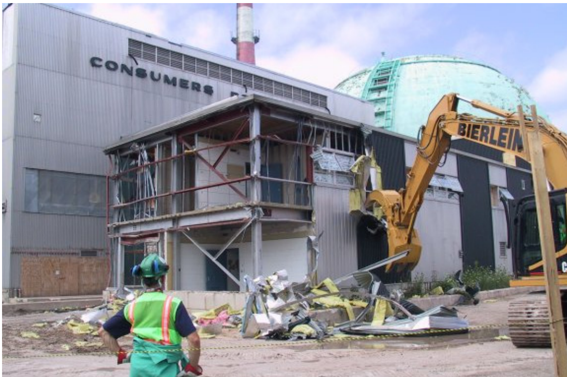
Demolition begins on the former administration building
