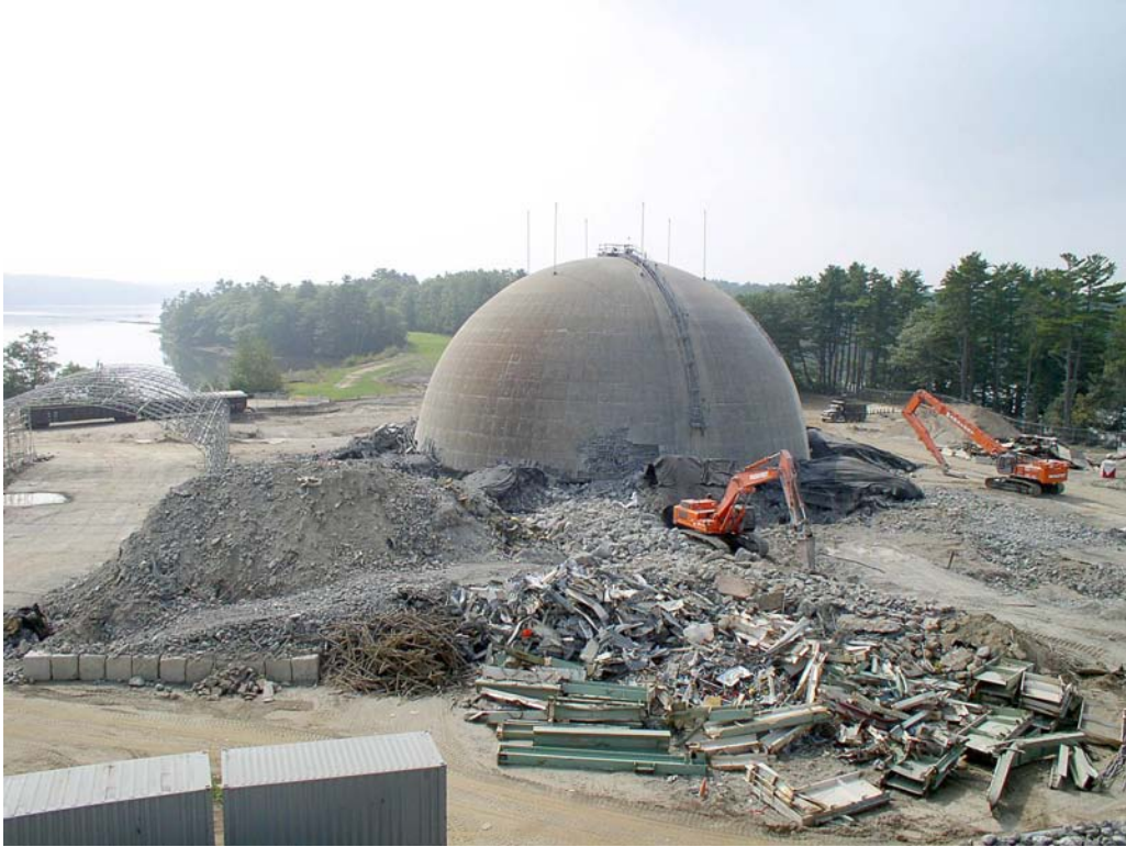
Containment After Demolition
