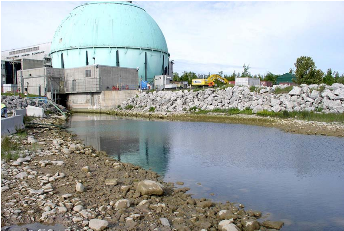
The discharge canal is shown before remediation efforts
