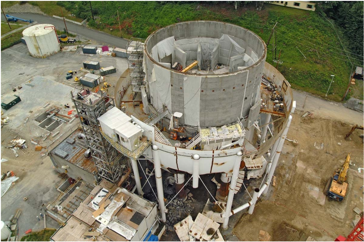
View of Reactor Support Structure – June 2004
