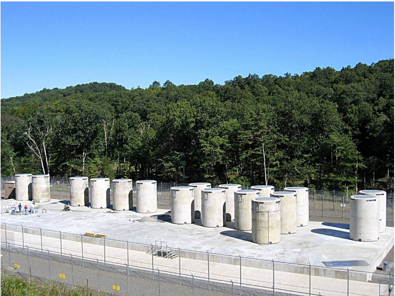
Connecticut Yankee ISFSI with 17 Vertical Concrete Casks
