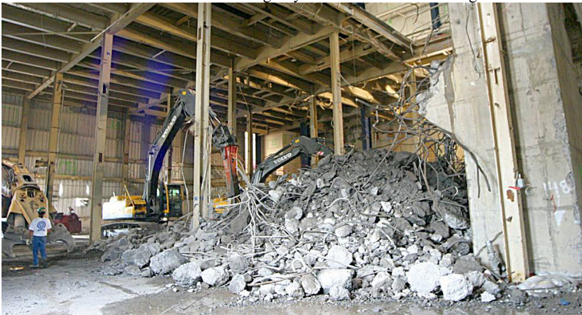
Demolition of the Turbine Pedestal
