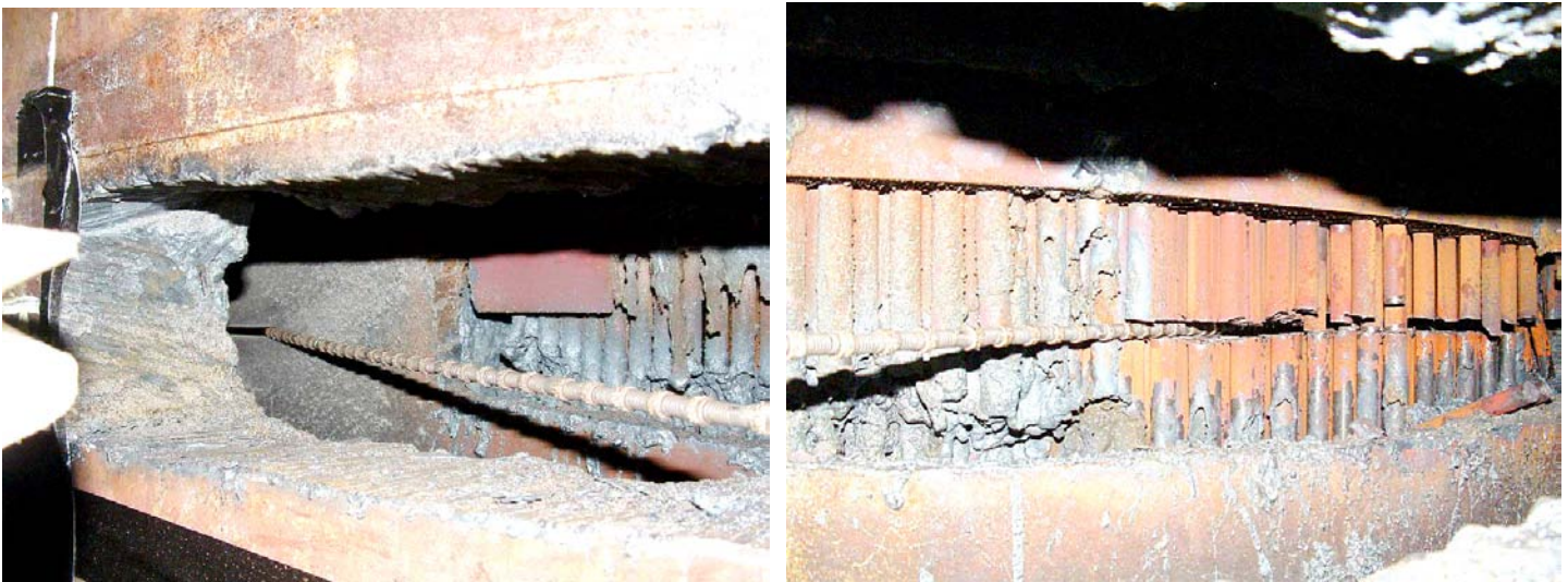
Steam Generator being cut with diamond-wire saw through hole in shell
