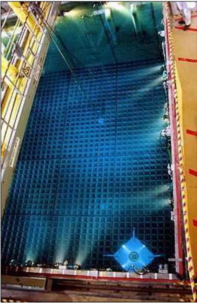
Spent Fuel Pool – before
