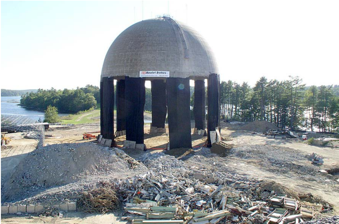
Containment Before Demolition
