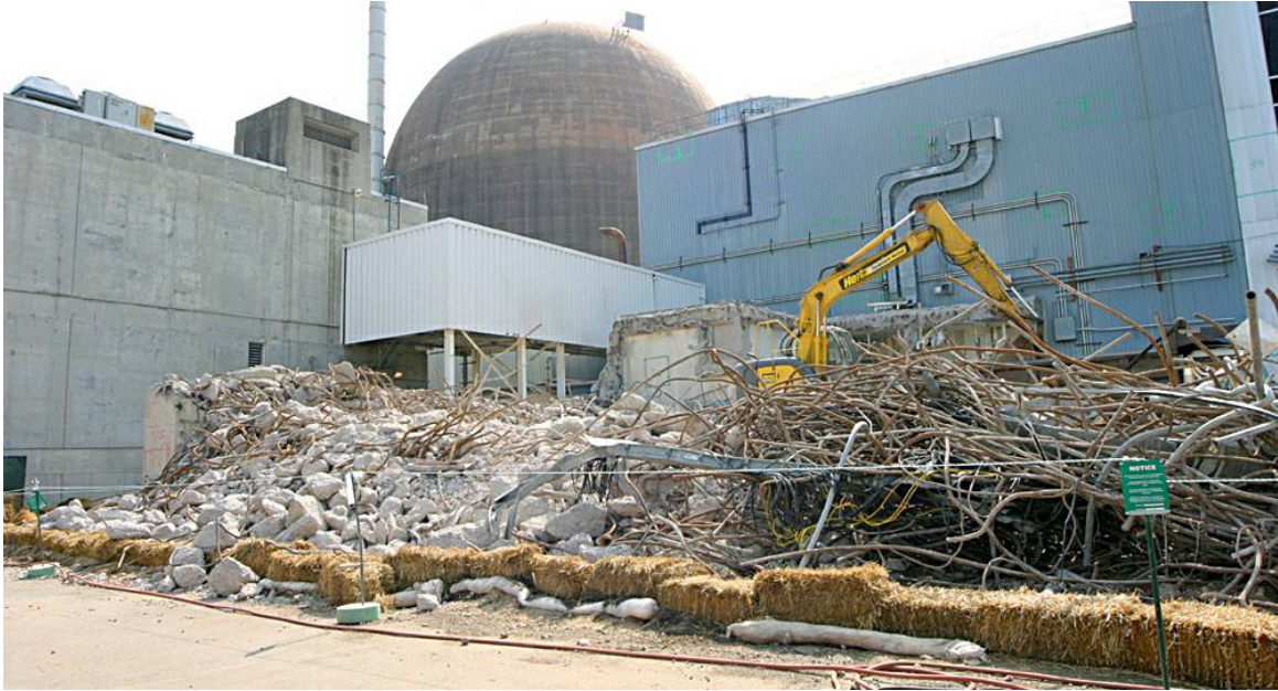
Demolition of the Emergency Diesel Generator Building
