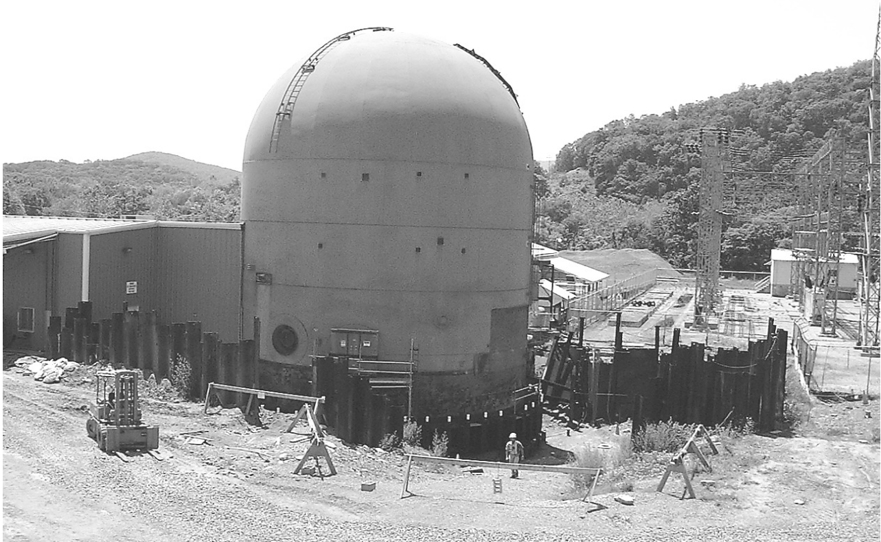
Saxton Before Dome Removal
