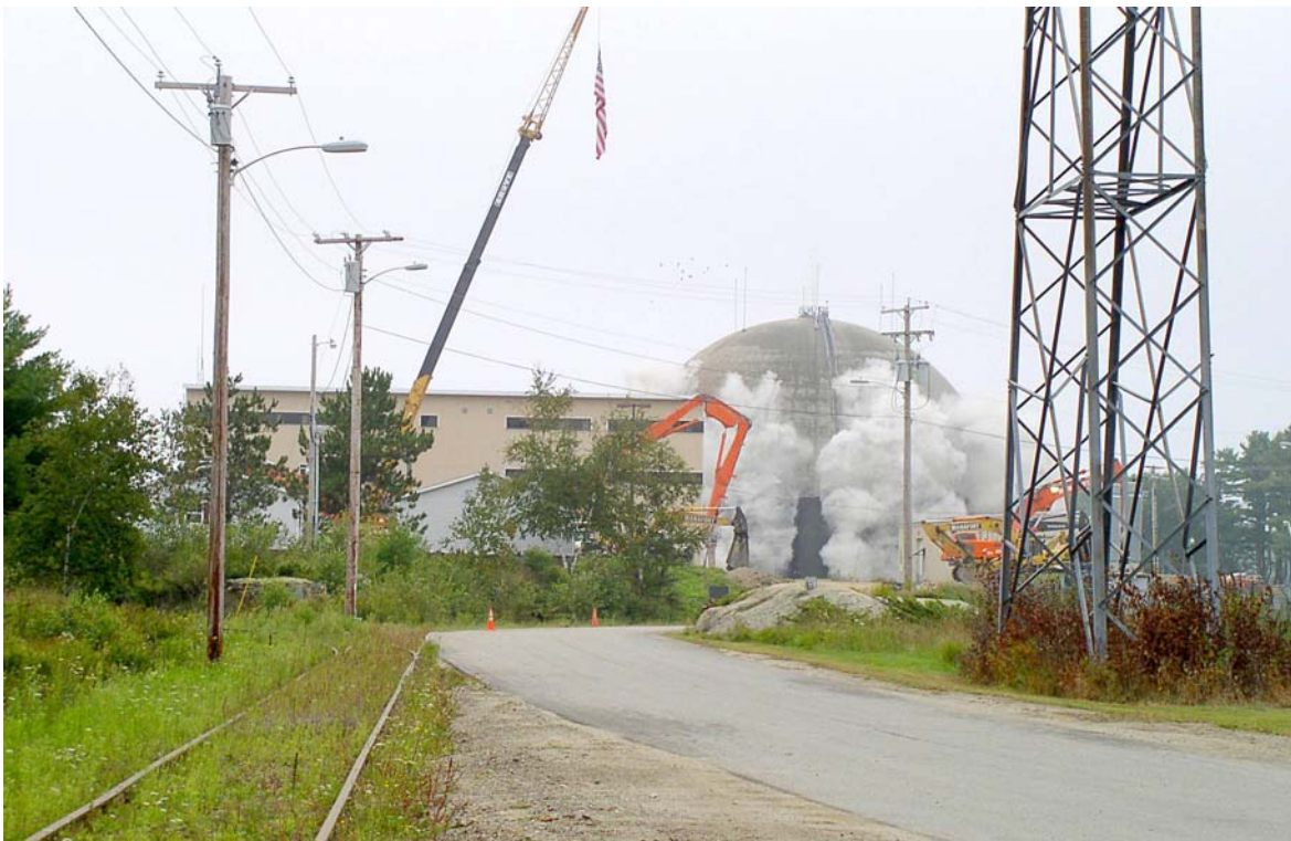
Containment During Demolition
