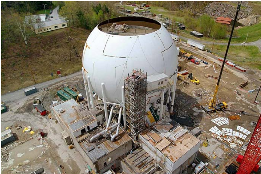
Aerial View of Vapor Container – May 2004
