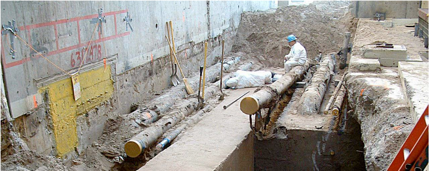
Underground Pipe Removal
