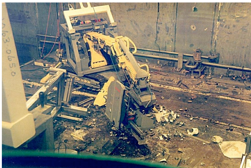
Dismantling using the Brokk
