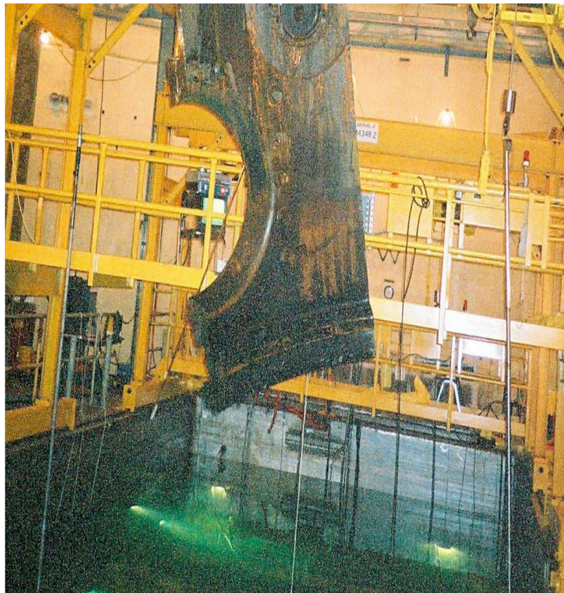
Vessel Internals – Piece of Core Support Shield (Class A)
