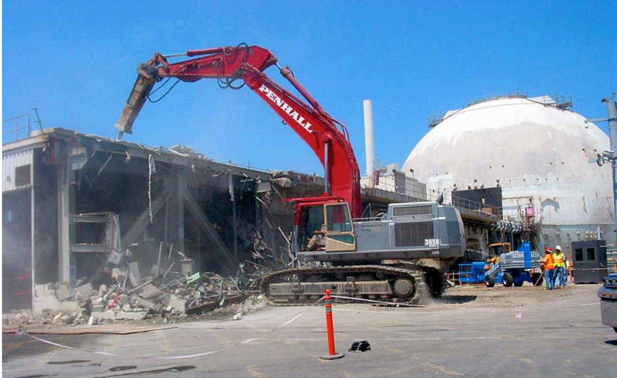
SONGS 1 Turbine Deck Demolition
