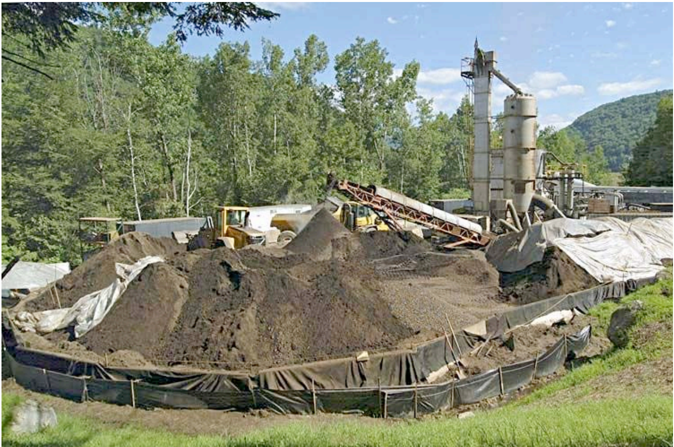
Soil Remediation with Thermal Desorption
