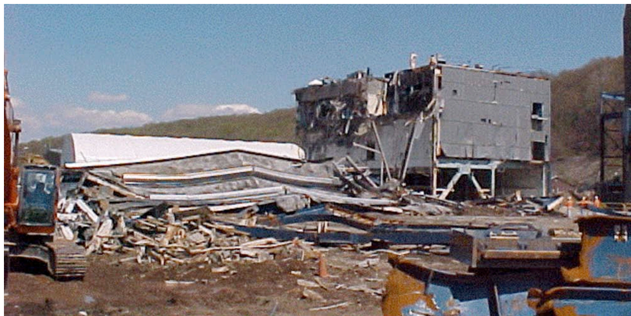
Turbine Building Demolition
