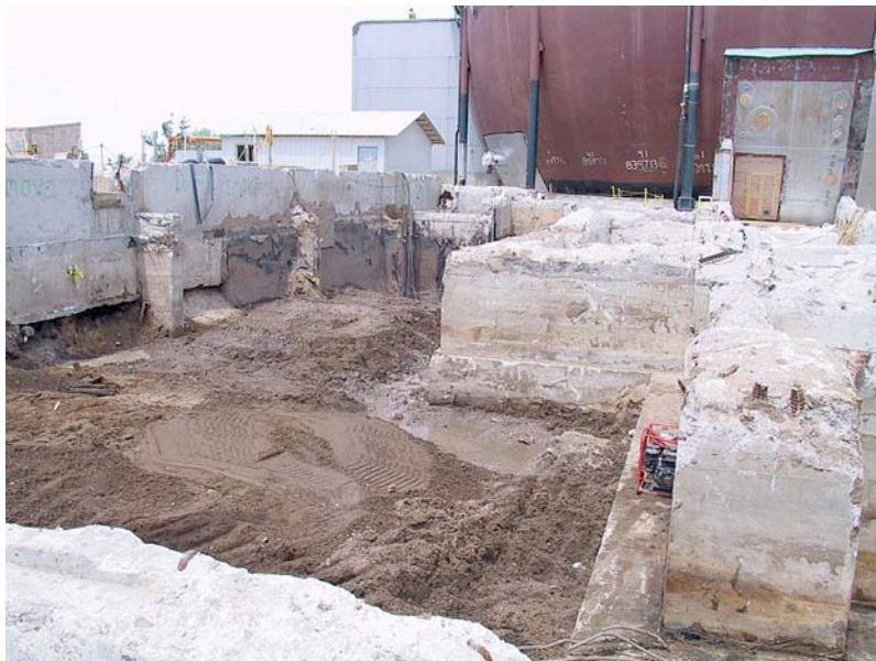
Turbine Building Foundation Removal
