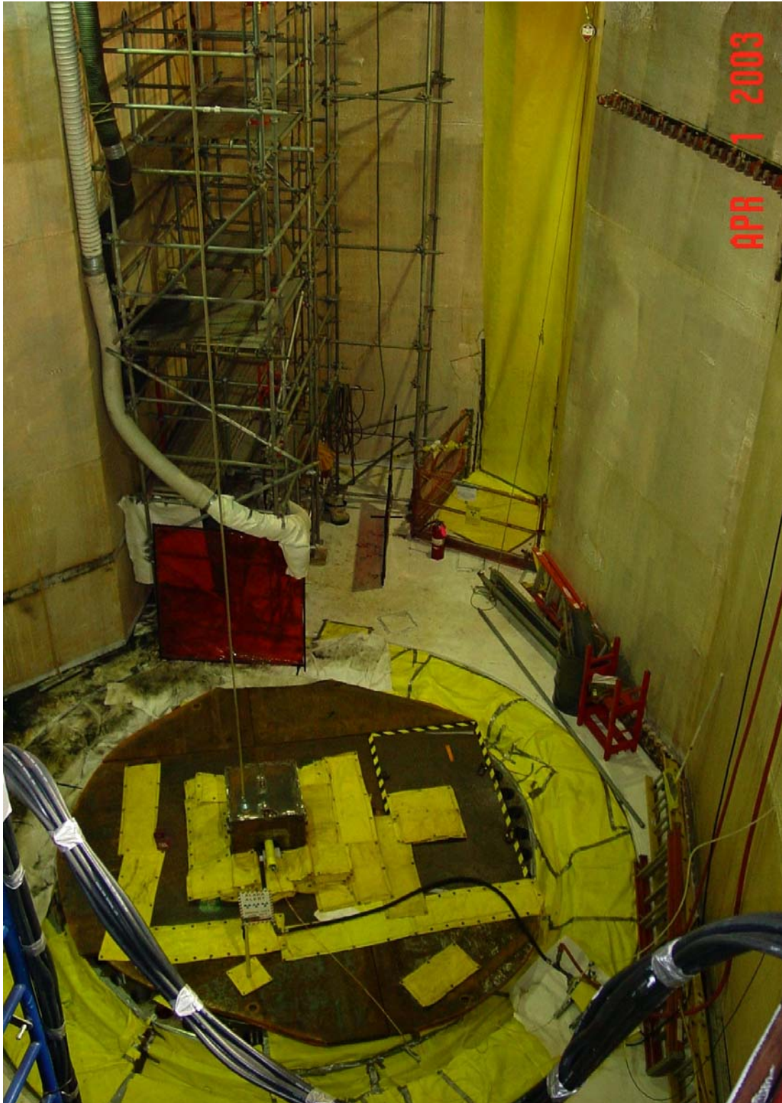
Cavity Prep Work after Drain Down
