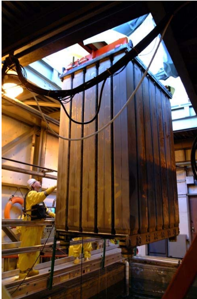
Fuel Storage Rack Removal from Spent Fuel Pool
