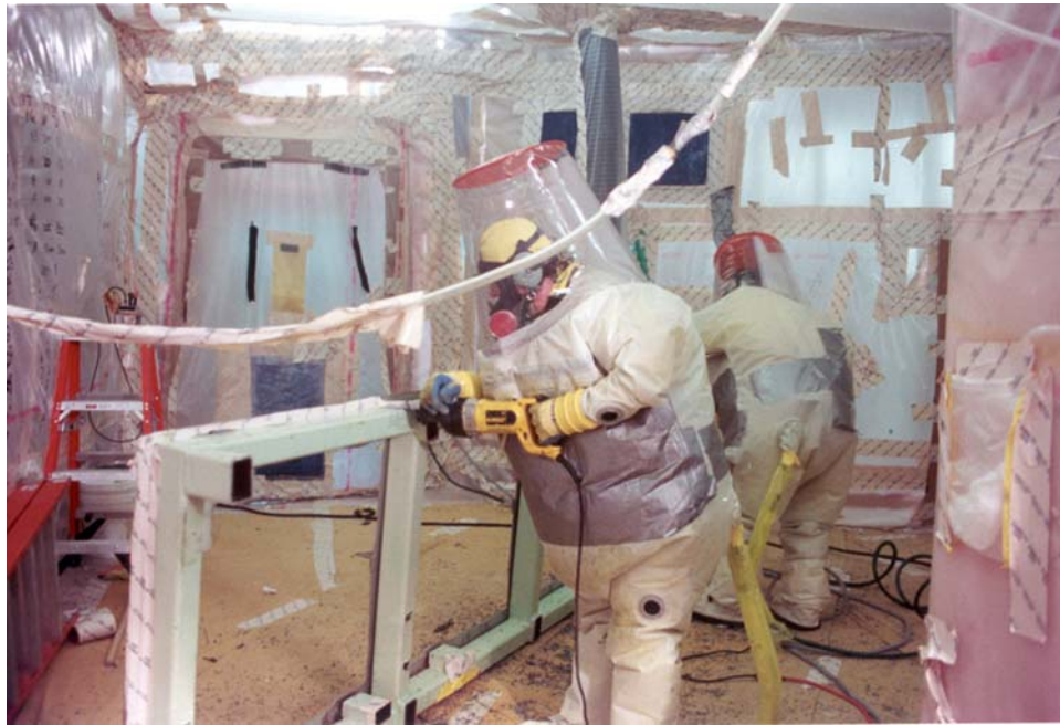
Steelworkers dismantling the last, highly contaminated glovebox in Building 771..
