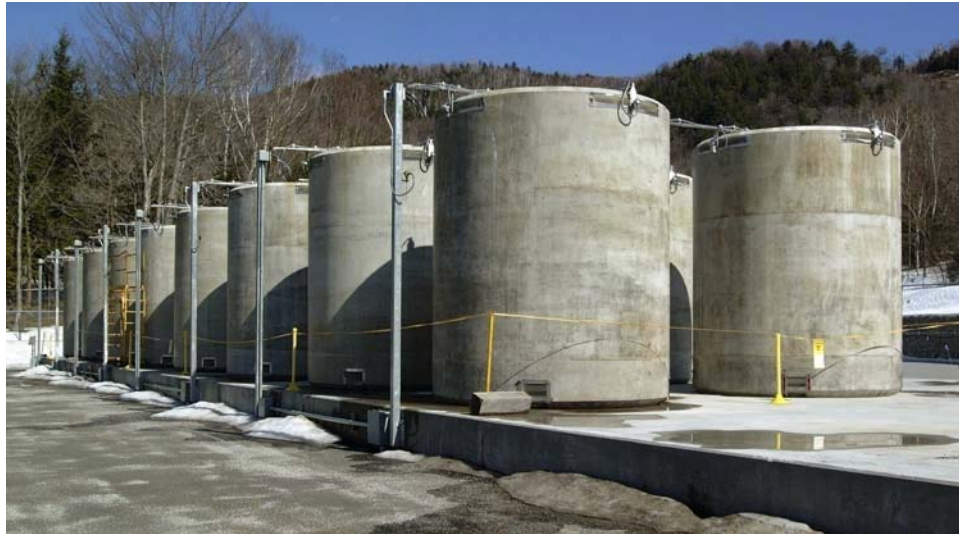
Fourteen Loaded Vertical Concrete Containers on Fuel Storage Pad
