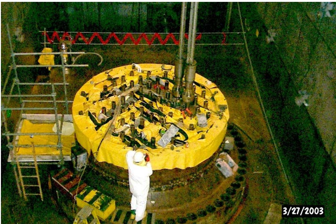
Removing Control Rod Drives Prior to Head Removal
