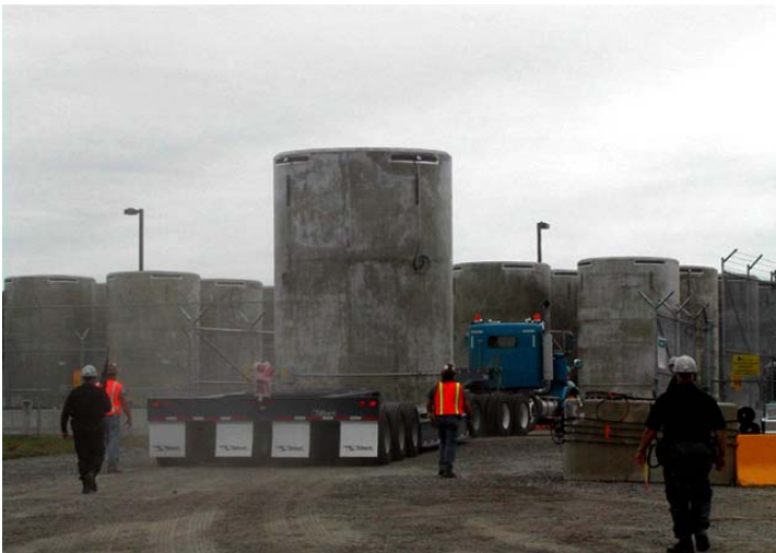
First loaded Vertical Concrete Cask to ISFSI
