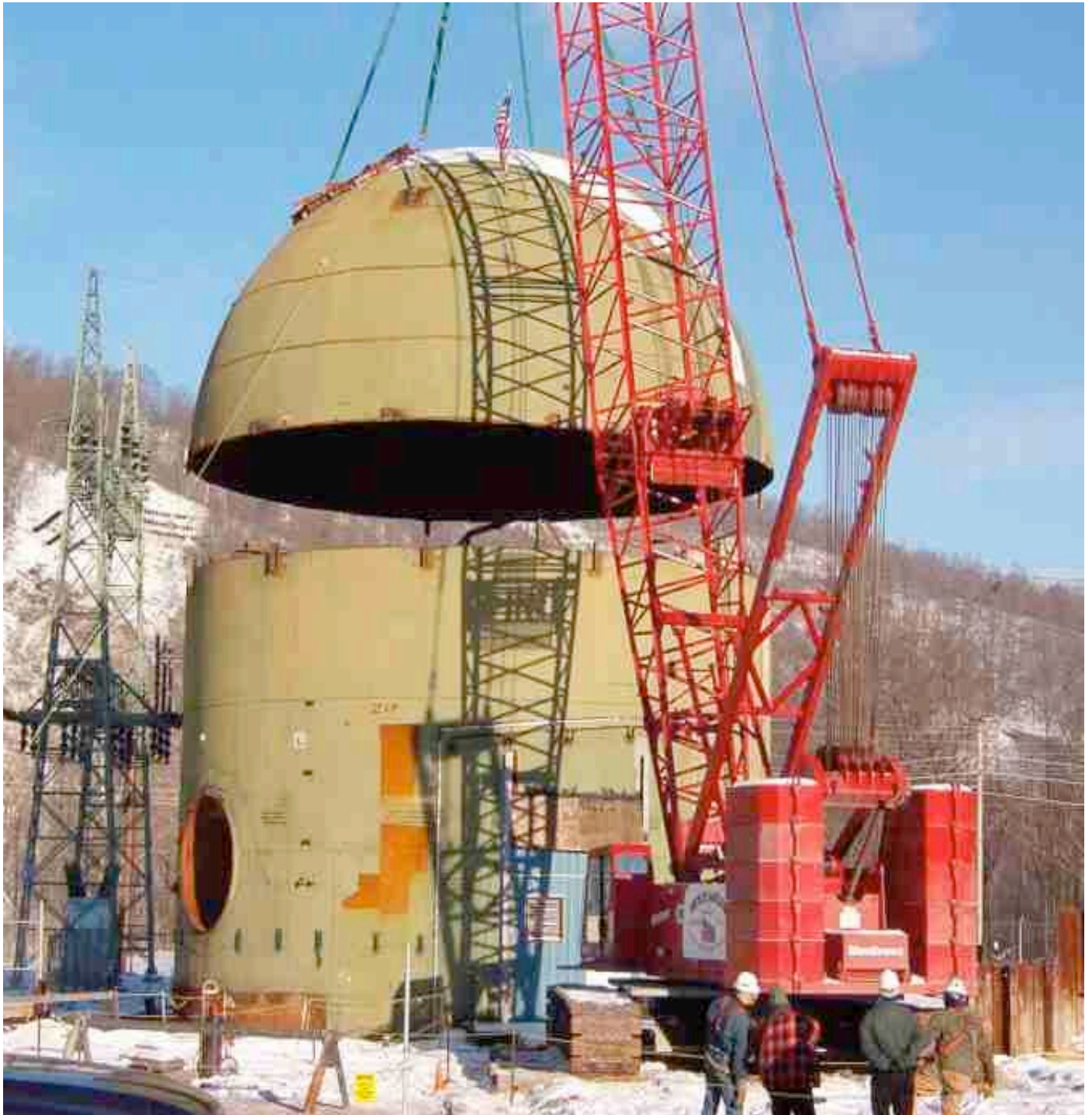
Containment Vessel Dome Removal
