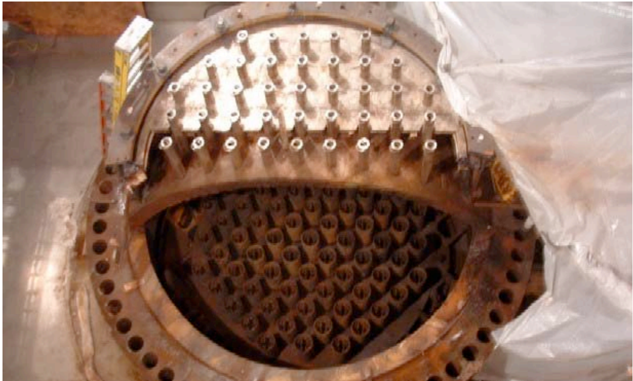
Reactor Vessel Head on Vessel after 1 st Cut
