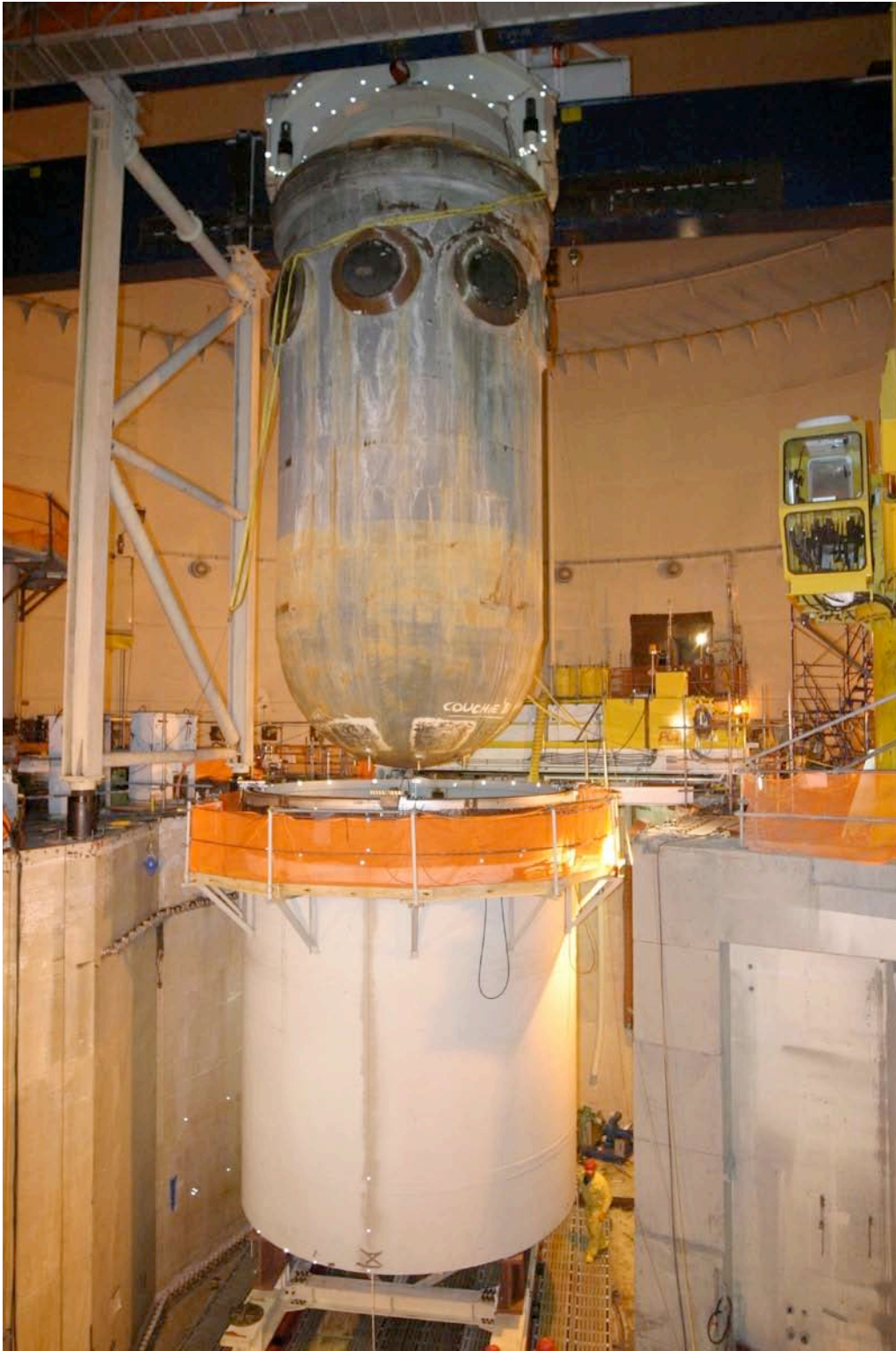
Placing the RPV in the Lower Section of the Shipping Container
