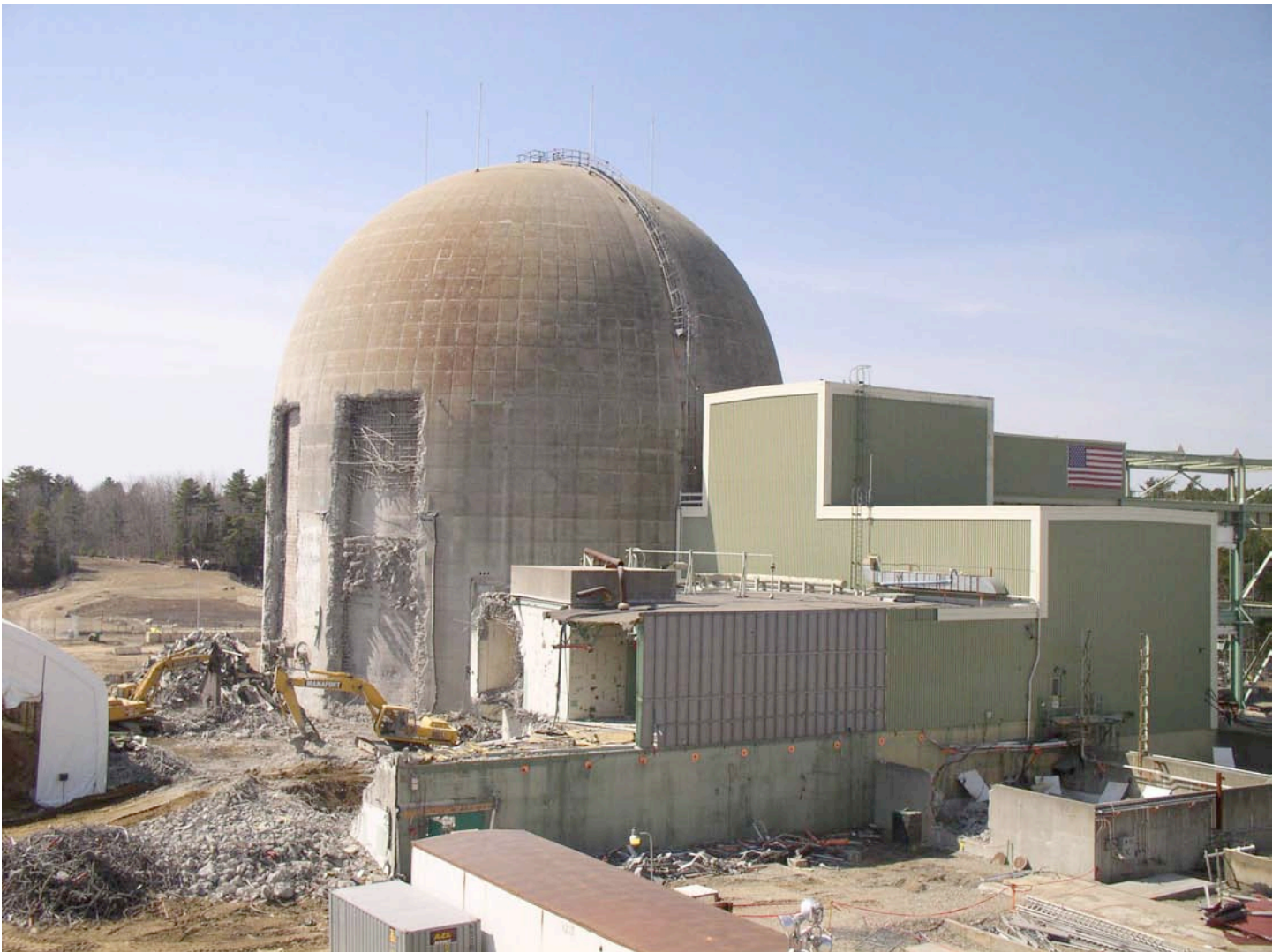
Exterior Containment Demolition
