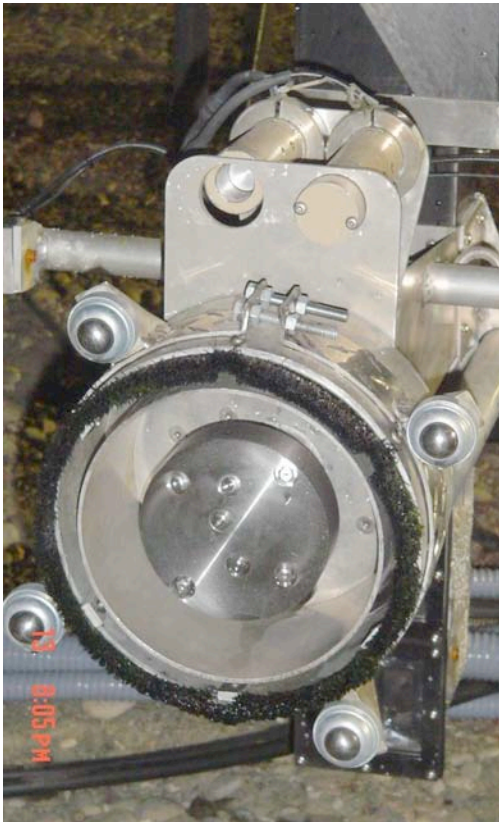
Hydrolazing Equipment to Reduce Contamination on Walls Prior to D&D
