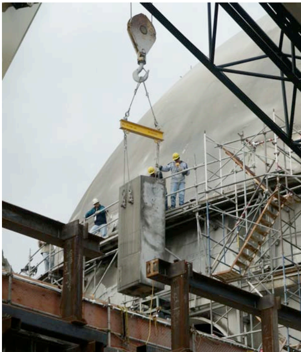
Demolition/Removal of Sphere Enclosure Bldg By Conventional Means
