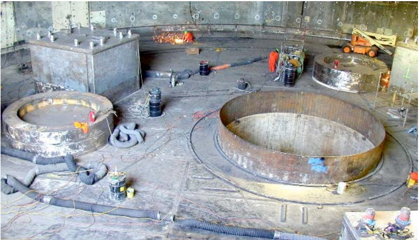
Interior Containment Remediation
