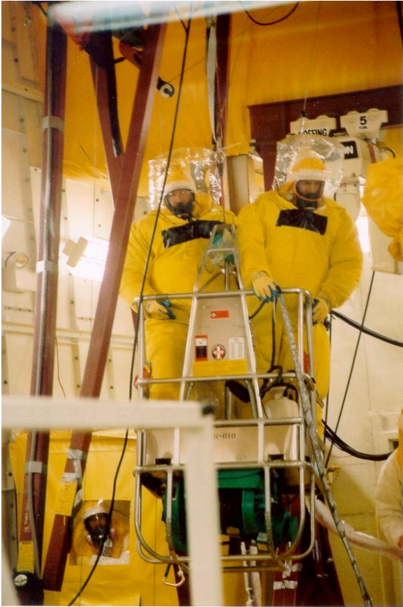
A Spider basket is used to raise and lower Operators into Extraction Cell-2.
