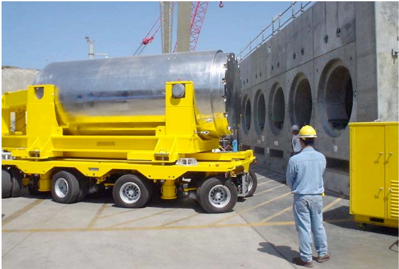
Fuel movement of Unit 1 spent fuel from Unit 1 to the ISFSI
