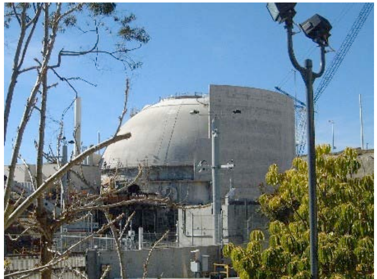
Containment Sphere Demolition
