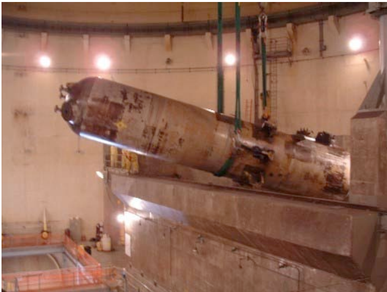
Pressurizer Removal
