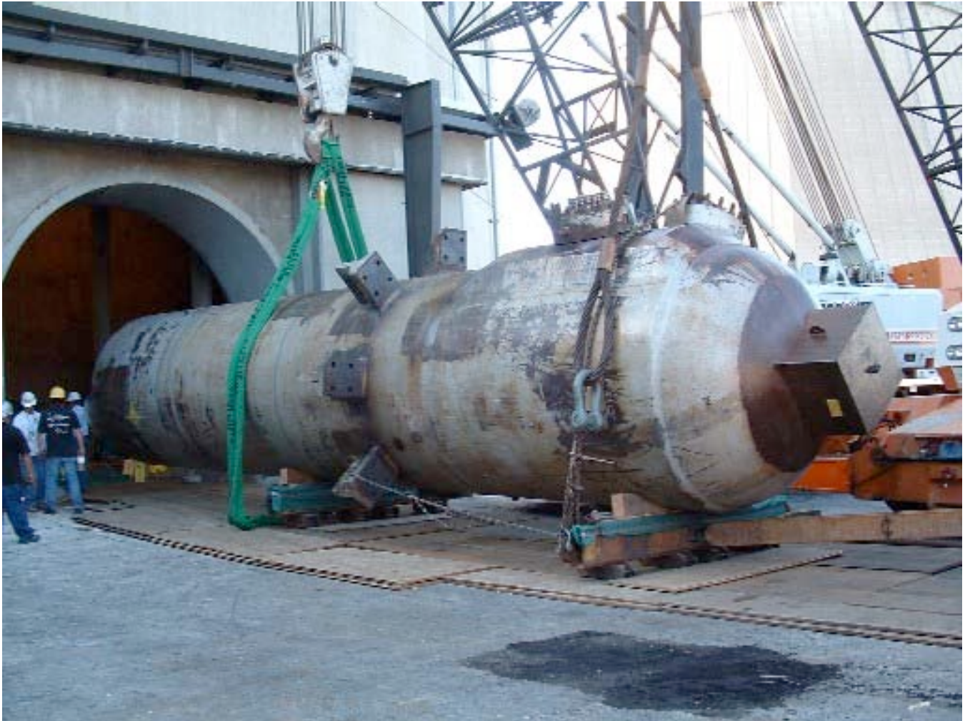
Removing the Pressurizer
