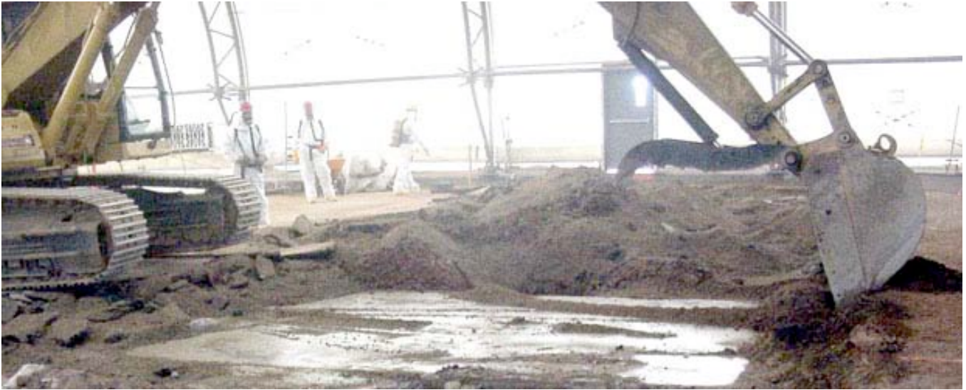
More than 32,000 tons of contaminated soil and asphalt were removed during the 903 Pad Cleanup
