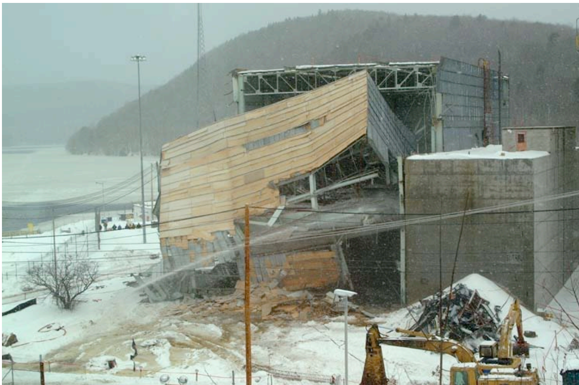
Turbine Building Demolition
