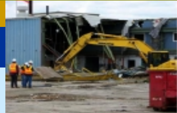
Maintenance Facility Demolished
