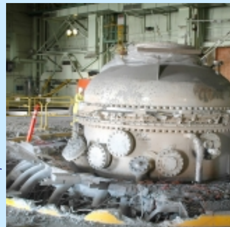
ETR Bioshield Demolition
