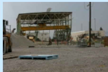
ETR Building Demolition
