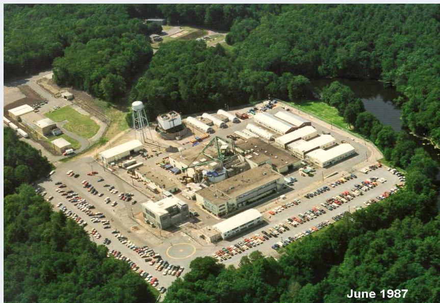
Before — The S1C Prototype Reactor Site and Support Facilities
