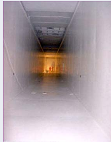
Figure 5 – Example: Cleanup of Decladding Conveyor Channel
