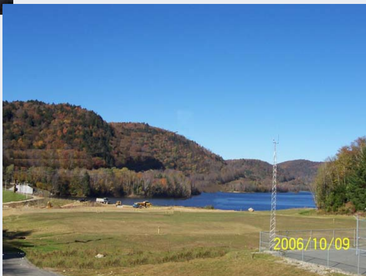
Views of the Yankee Rowe site after completion of physical decommissioning activities.
