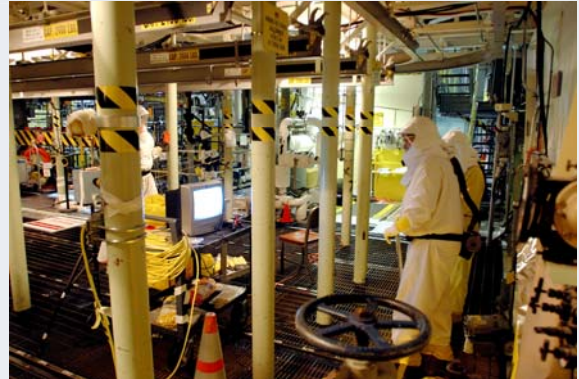
Fluor Hanford completed containerizing bulk sludge in the KE Basin in the Fall of 2006.
