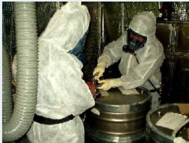
Heavy water retrieval work at Fugen.
