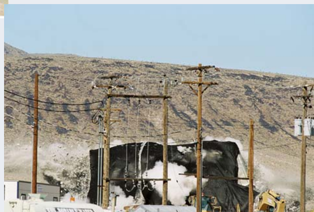
Shield wall during controlled explosive demolition.
