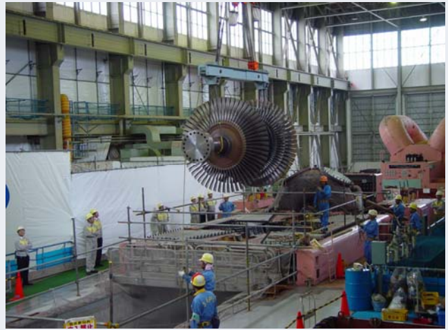
Removal of low pressure turbine at Tokai.
