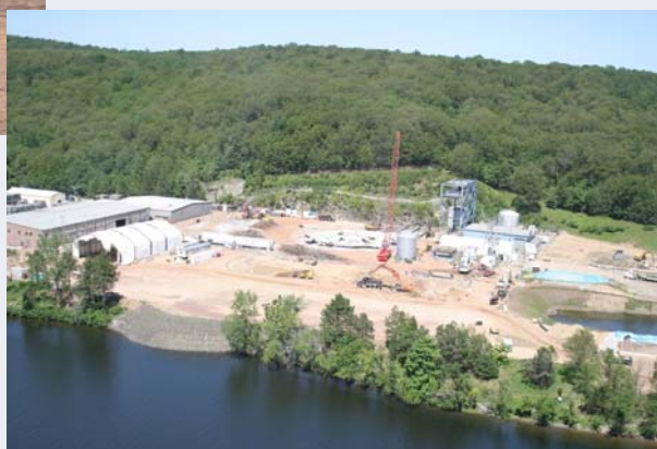
Aerial view of the Connecticut Yankee site – August 9, 2006
