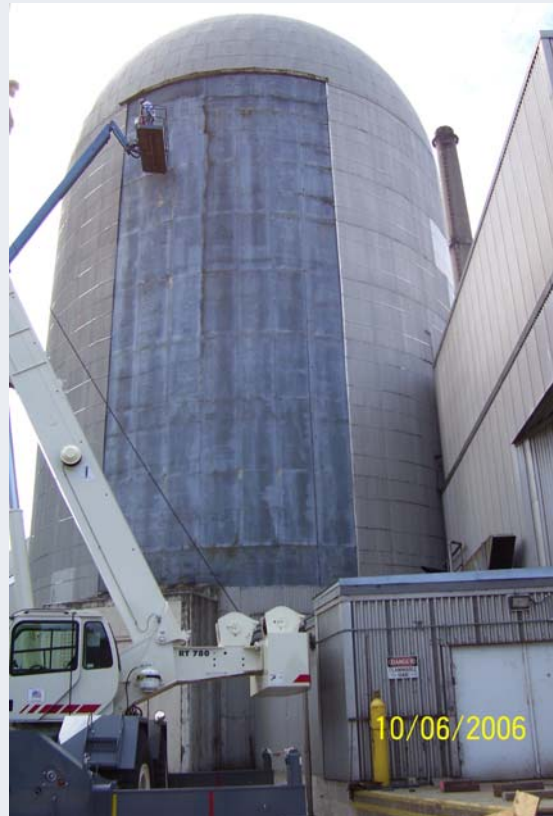
Reactor Building siding removal
