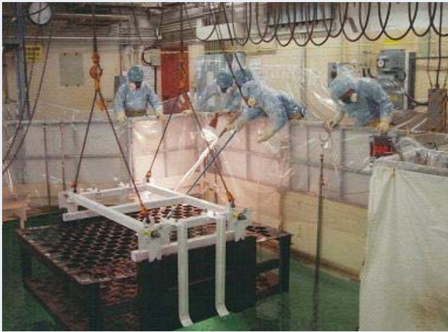
Spent fuel storage rack cleaning at Tokai.
