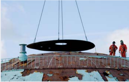
Dismantlement operations at Big Rock.
