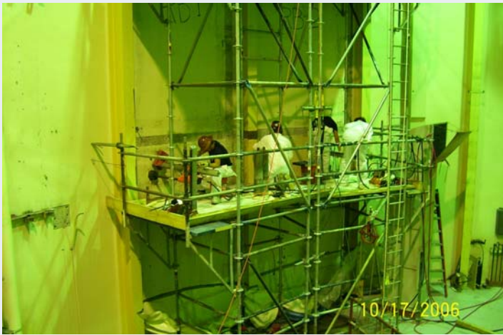
Drilling rigging holes in the Reactor Building
