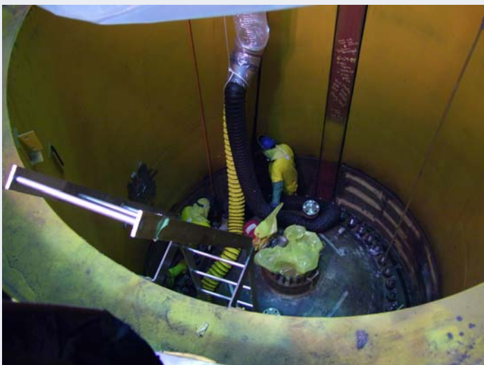
Insulation ring cutting
