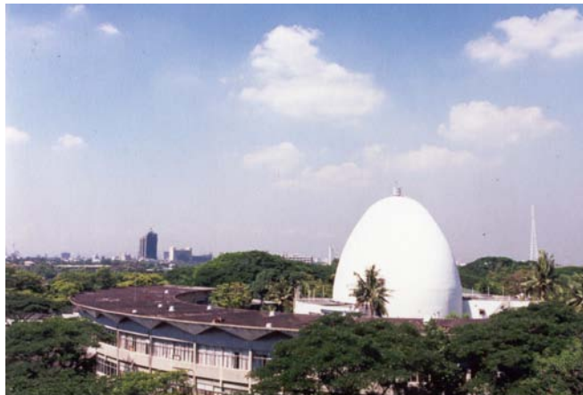
Figure 3: Dome of the Philippines Research Reactor
