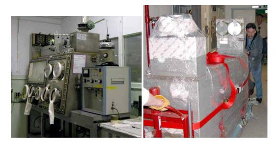
The D&D workers at the Plutonium Finishing Plant are making progress within the 234-5Z Building, a former plutonium processing facility. Glovebox removal continues ahead of schedule so that demolition of the facility can be accelerated.
