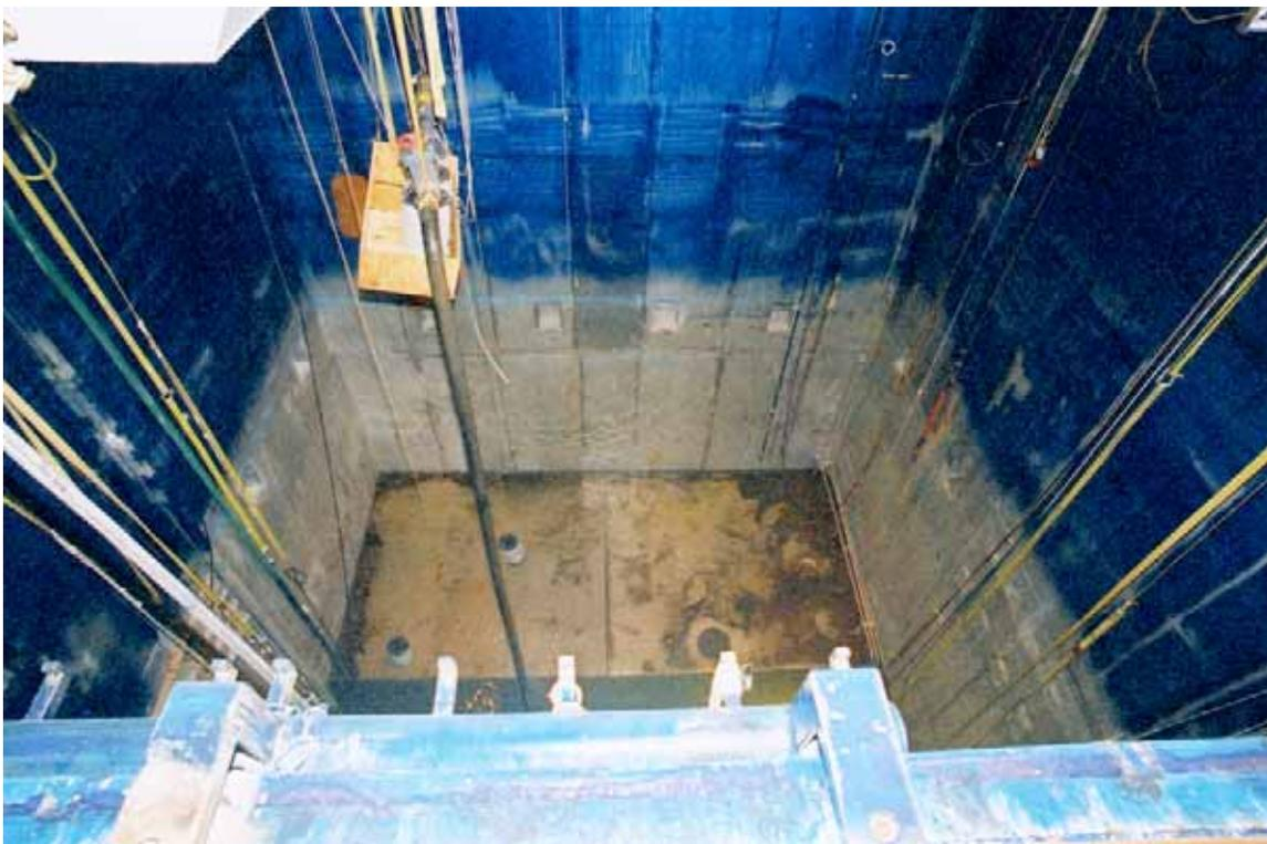
**49 foot Level, Cask Loading Pool Being Emptied (Blue Area is fixative for contamination)**
