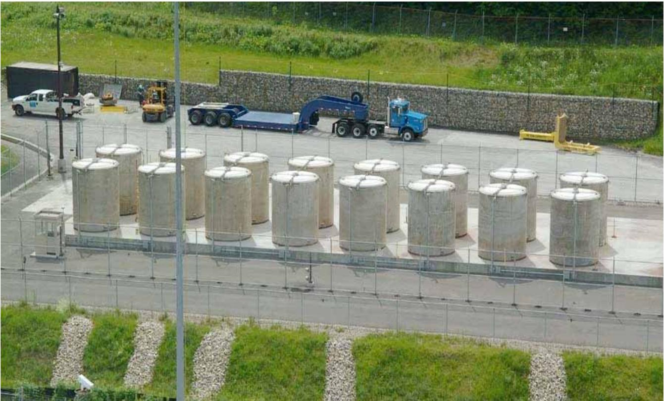
**16 Loaded Casks in the ISFSI, 15 with fuel, 1 with GTCC**
