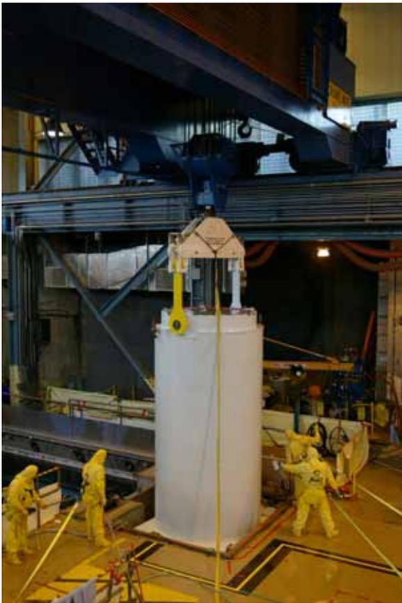
**MPC Removal from Cask Load Pit**
