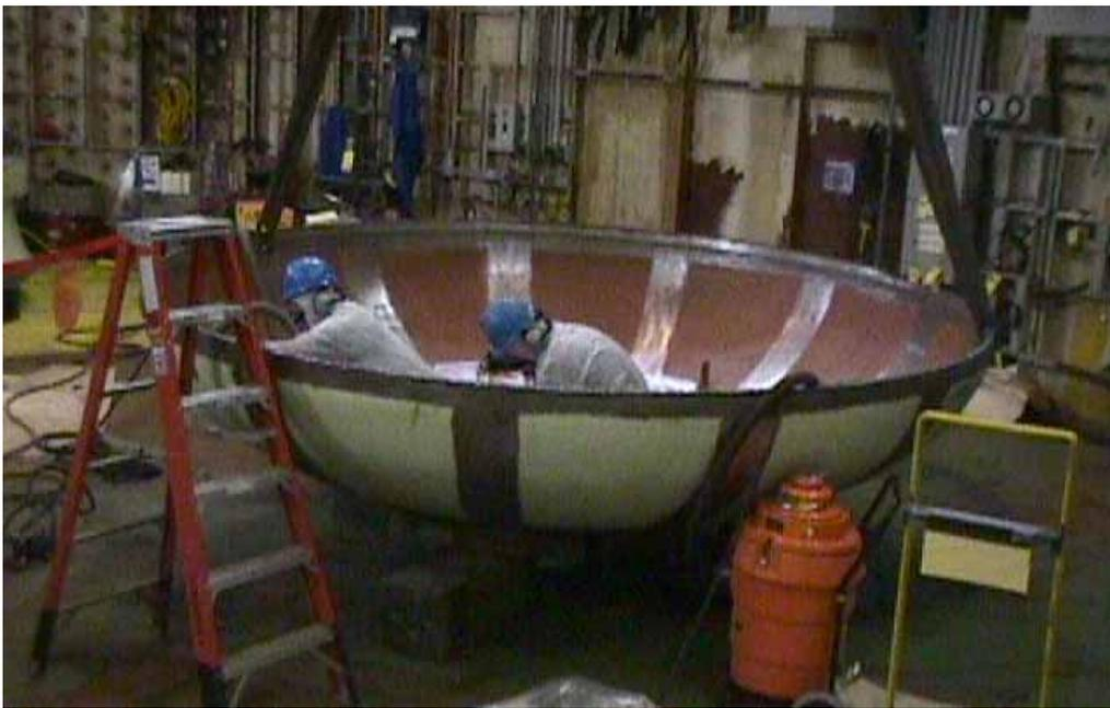
**Abating Paint from the Reactor Machinery Dome**
