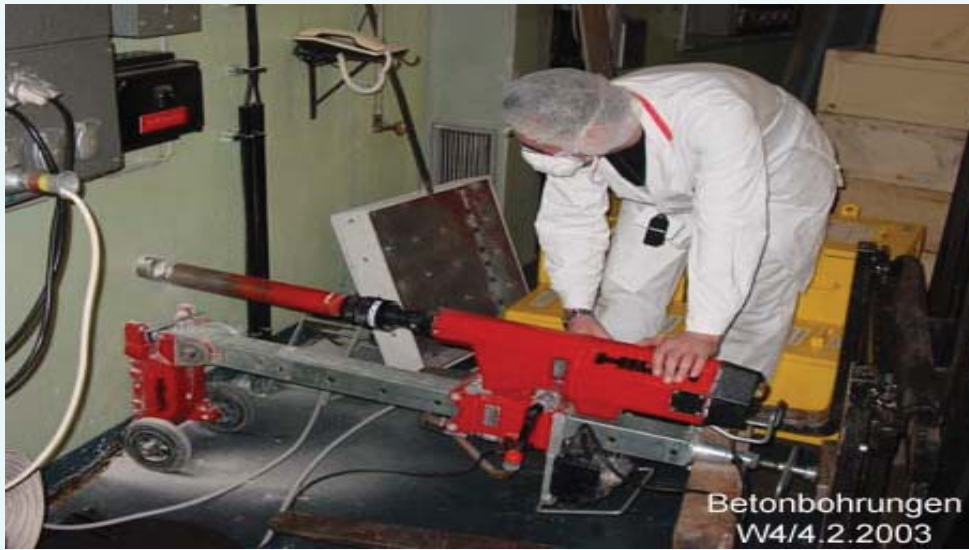
Fig 1 Core drilling tools at ASTRA reactor decommissioning project, Seibersdorf, Austria
